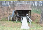
Romania, Watermill, with Vertical Overshot Wheel and Two Gear Transmission, originally from Rogojelu, Cluj County, reconstructed and presented in ASTRA Museum, Sibiu, as the work with the index MA57.
